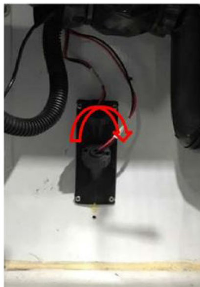
Figure 10.5 Supply Air Sensor Removal
