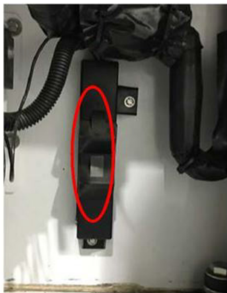
Figure 10.5 Supply Air Sensor Removal
